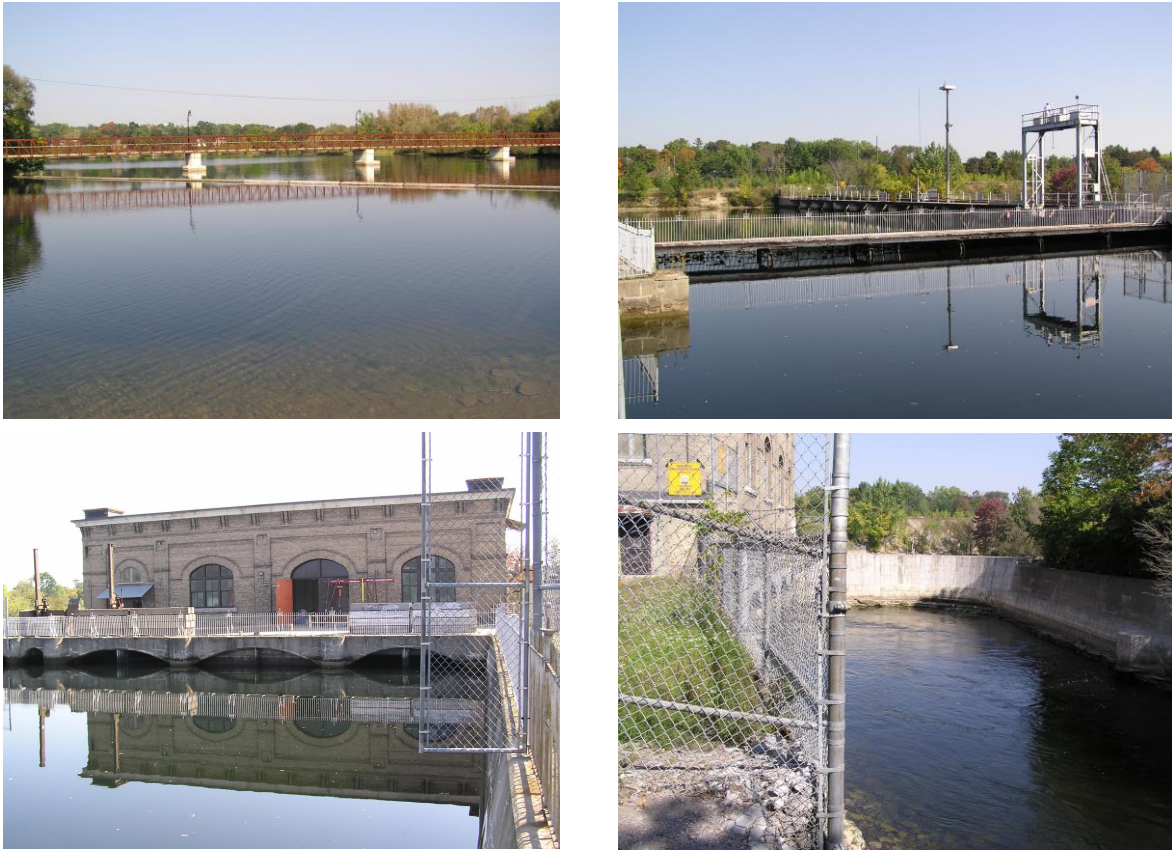
Figure 3: Photos of the London Street Generating Station and Control Dam. The top photos are of the control dam, with the separate head canal shown in the top right photo. The bottom left photo shows the generating station viewed from upstream. The separate tailrace is shown in the picture on the bottom right.
