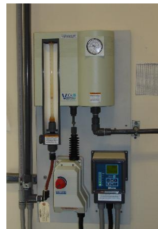
Zebra mussel chlorine dose modulator
