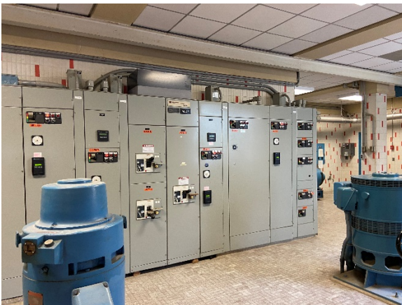
Figure 13: Electrical Panel and MCC
