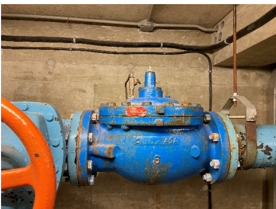
Figure 17: Pressure reducing valve
