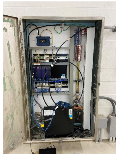
Figure 22: SCADA and electrical cabinet
