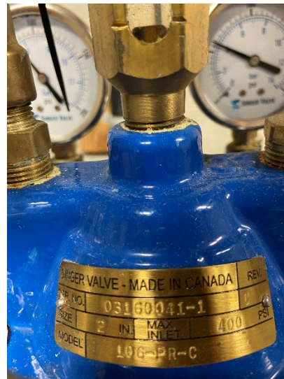
Figure 16: Label on 2" pressure reducing valve
