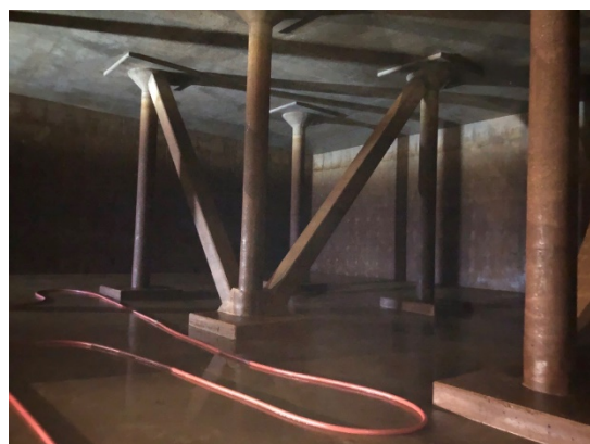
Figure 65: Chlorine is fed through the red hose
