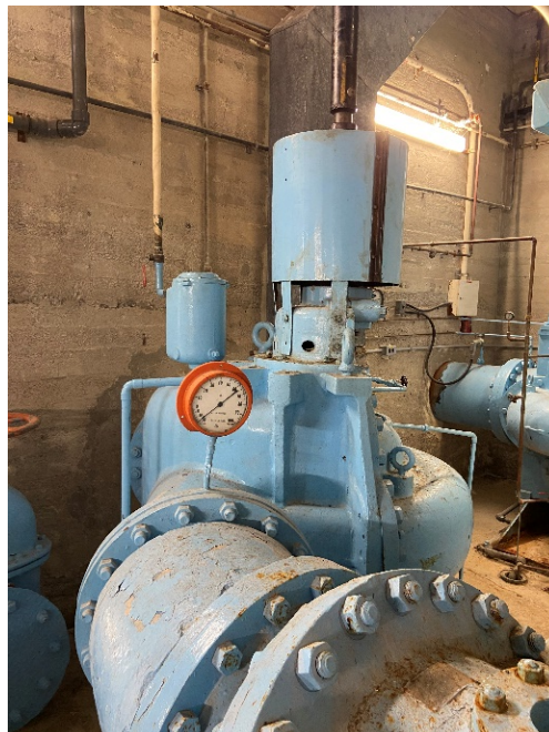
Figure 4: Diesel Powered Low Lift Pump #3
