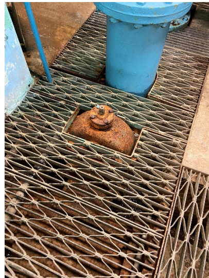
Figure 48: 12" gate valve
