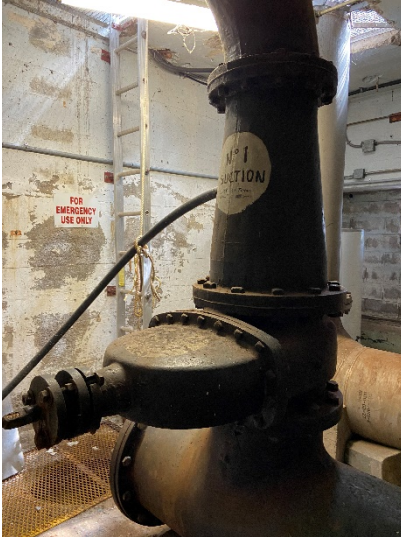
Figure 1: Pump 1 18" suction gate valve
