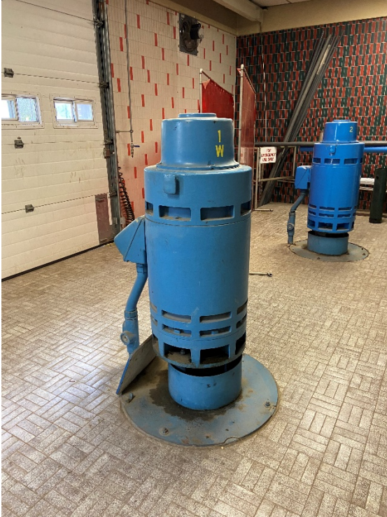
Figure 11: Backwash Electric Motor #1
