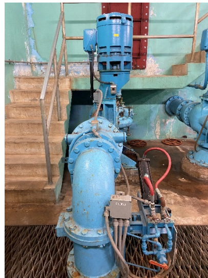
Figure 14: Pump 1 and butterfly valve
