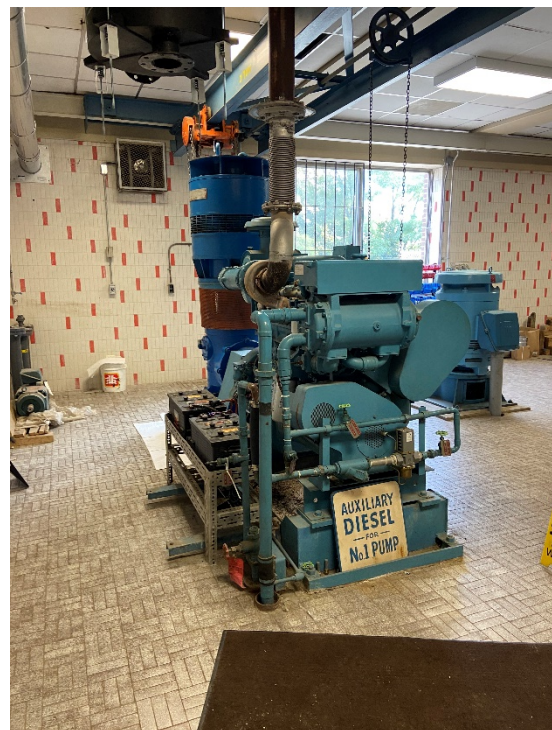
Figure 8: Pump #1 Diesel Motor
