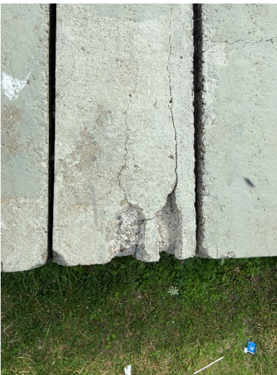
Figure 3: Cracks in concrete roof
