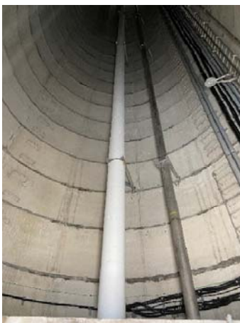
Figure 5: 12" feed pipe
