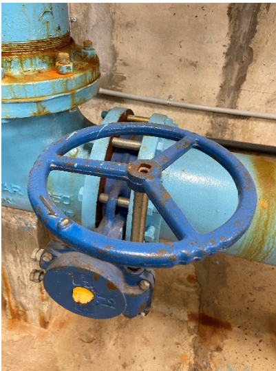
Figure 27: Discharge butterfly valve of pump 3 and pressure reducing valve
