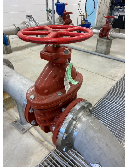
Figure 2: 8" suction gate valve on pump 1
