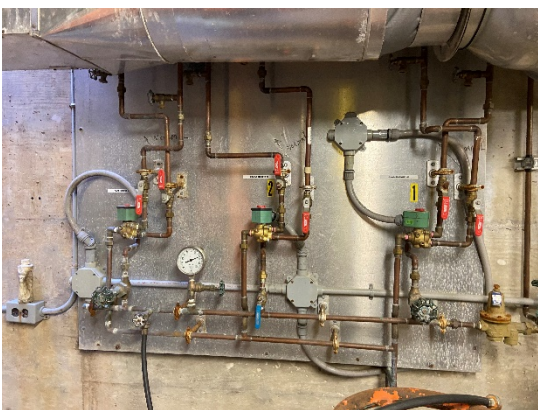
Figure 15: Automatic valve controls
