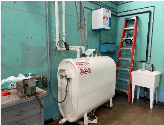
Figure 49: Pump 4 motor fuel tank
