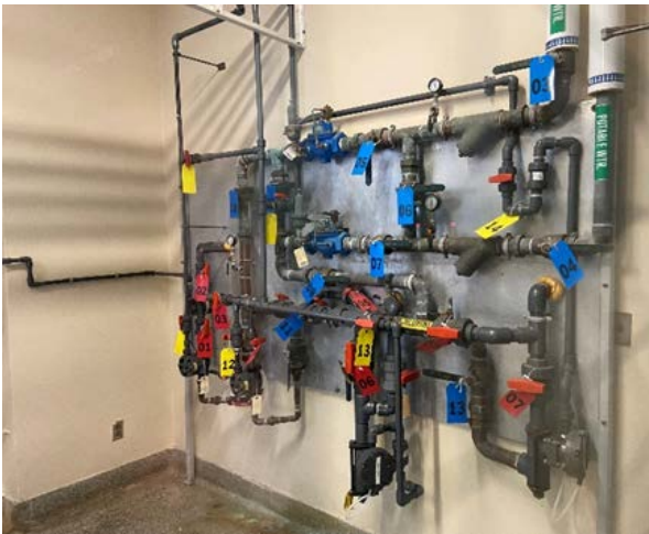
Figure 5: Chlorine Zebra-Mussel Control, Pre and Post Injectors
