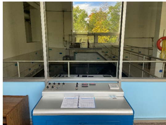
Figure 8: Filter Bed #7 and Controls
