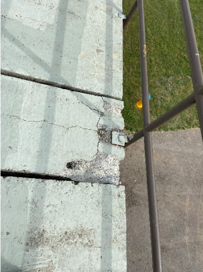
Figure 1: Cracks in concrete roof
