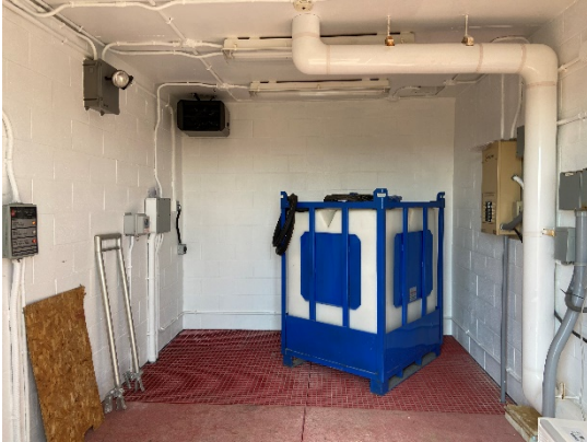
Figure 1: Chlorine tank in bricked building
