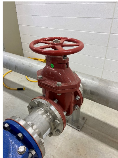
Figure 6: 6" discharge gate valve on pump 1
