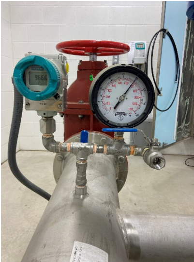
Figure 13: Discharge pressure gauge (Zone 3)
