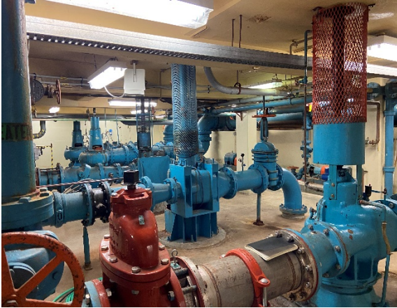
Figure 1: High Lift Pumps at Water Treatment Plant
