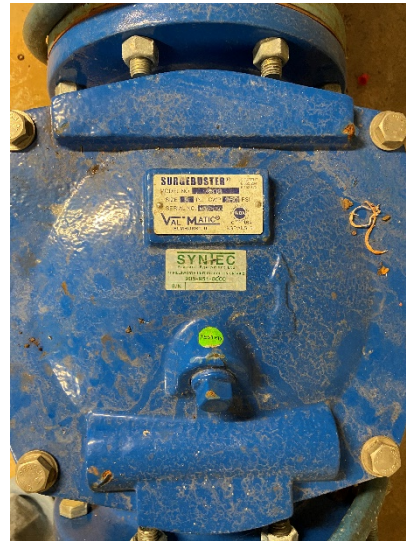
Figure 14: Swing check valve on pump 3
