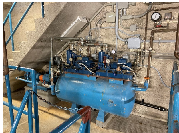
Figure 8: Vacuum Pumps, 1 duty, 2 standby
