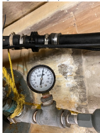
Figure 14: Suction pressure gauge
