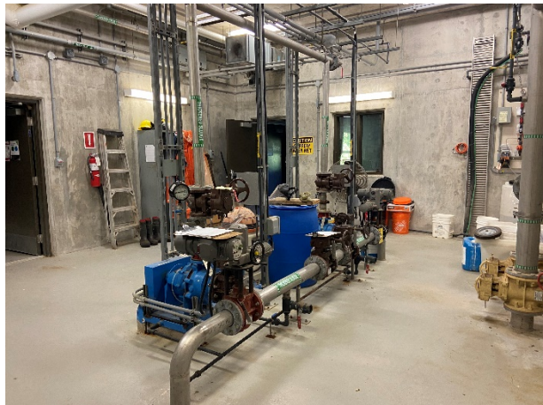
Figure 14: Thickened Sludge Pumps
