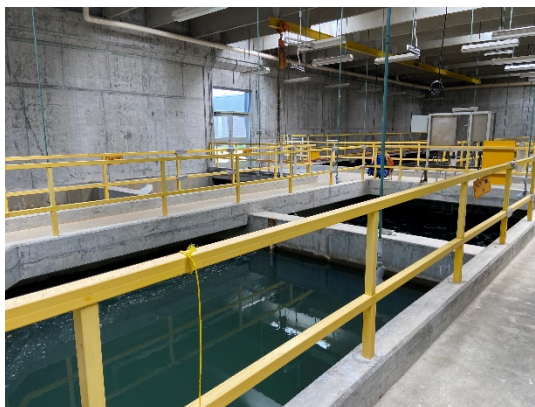
Figure 2: Floc Tank 6A(foreground) and 5C(background)
