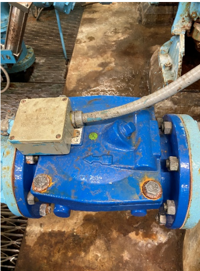
Figure 27: New check valve on pump 3
