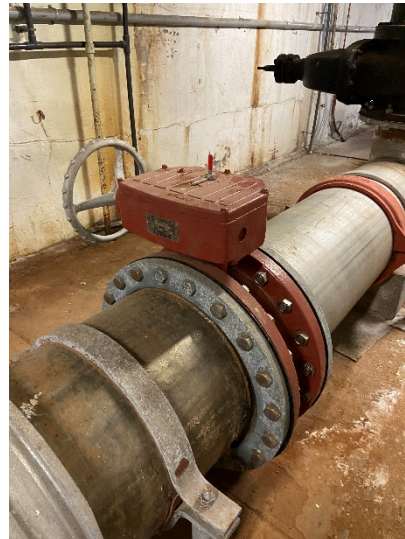
Figure 12: 20" butterfly valve
