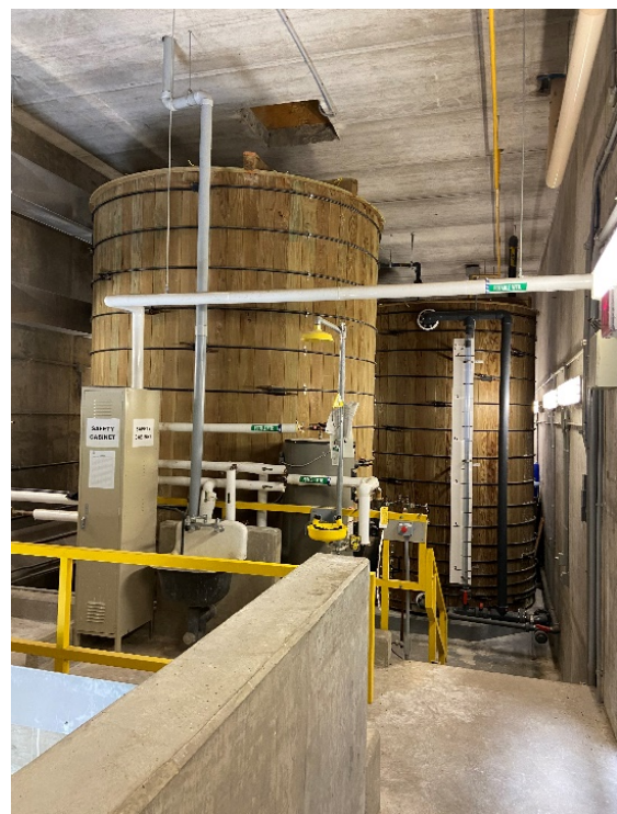
Figure 8: 3x 18,000L Coagulant Tanks
