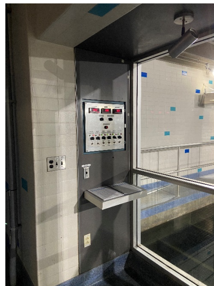
Figure 14: Filter Bed #10 Controls
