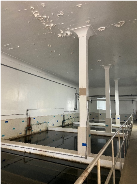
Figure 11: Filter Beds #3, 4, 5 and 6, ceiling in need of repairs
