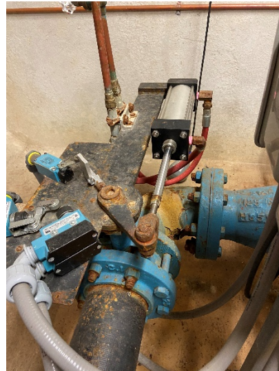
Figure 20: Butterfly valve on pump 2 (suction)
