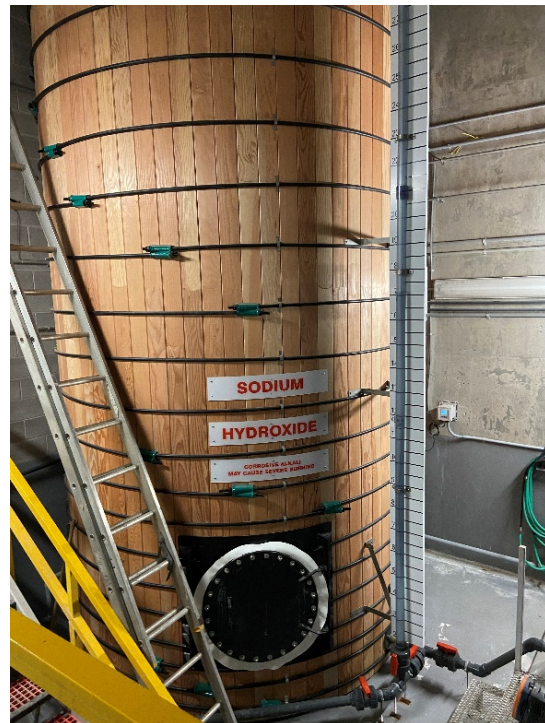
Figure 4: 30,000L Sodium Hydroxide Storage Tank
