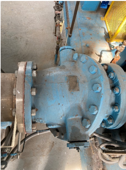
Figure 43: Pump 5 10" check valve
