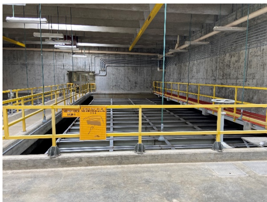
Figure 4: Sedimentation Basin 6
