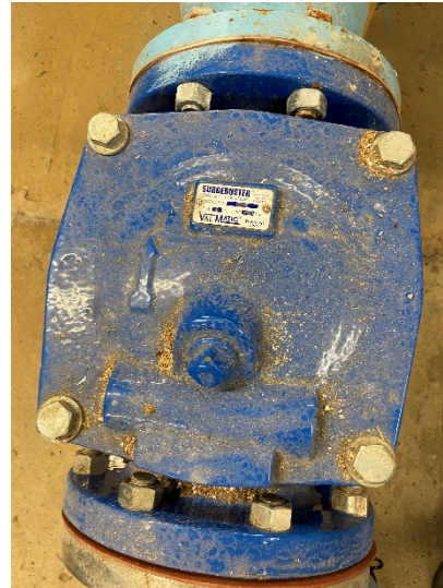
Figure 16: Check valve on pump 2
