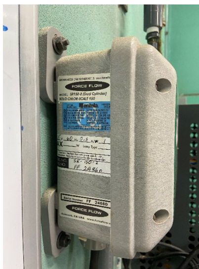
Figure 12: Label on chlorine scale
