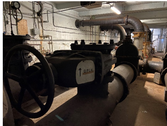
Figure 20: Gate valve on tee
