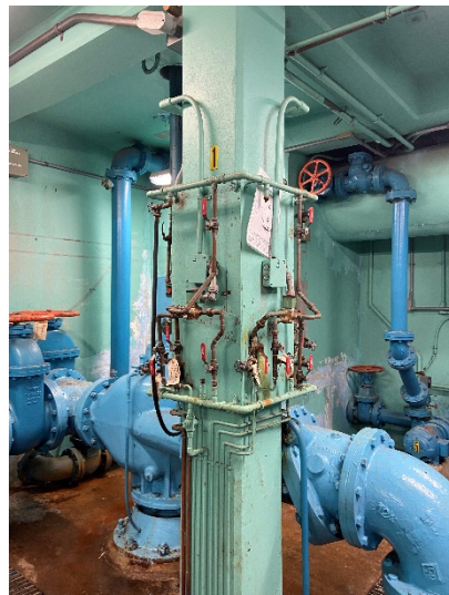
Figure 54: Butterfly valve controls
