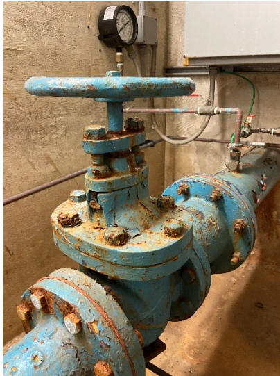
Figure 5: Gate valve on bypass
