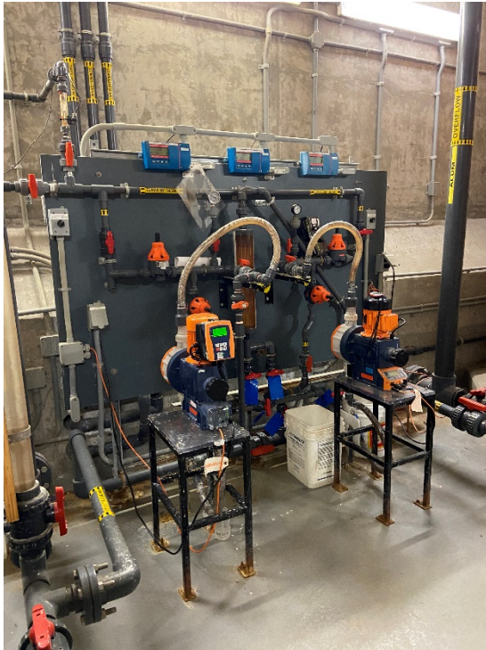
Figure 9: Coagulant Pumps, Piping and Controls
