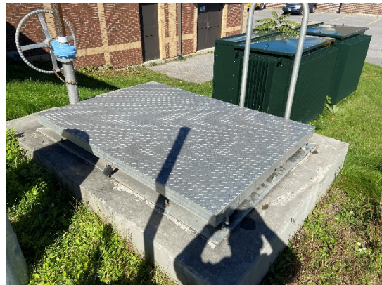
Figure 4: Access Hatch to Chlorine Contact Tank #1
