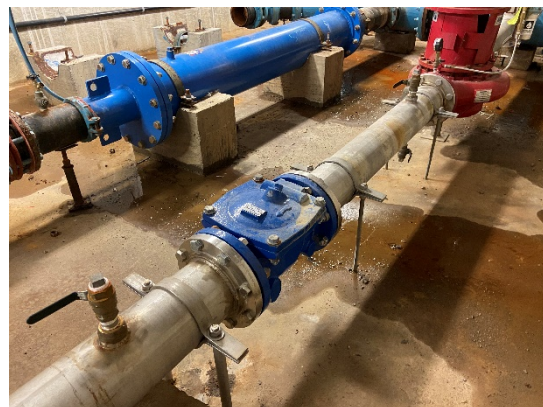
Figure 10: Check valve and inline pump
