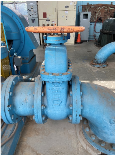
Figure 45: Pump 5 12" gate valve
