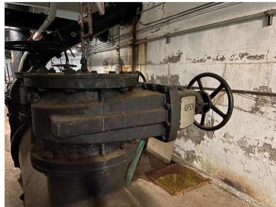
Figure 30: Disused gate valve
