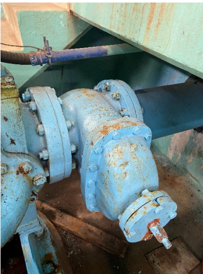
Figure 19: Gate valve on pump 1
