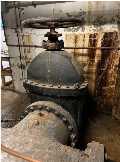
Figure 33: Darin 20" gate valve
