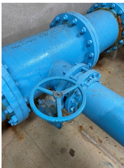
Figure 12: Butterfly valve on pump 2 (suction)
