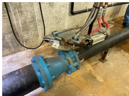
Figure 20: Reducer on pump 3
