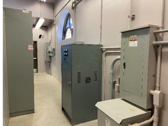
Figure 2: Switch Gear and SCADA
