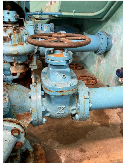
Figure 30: Gate valve on pump 3
