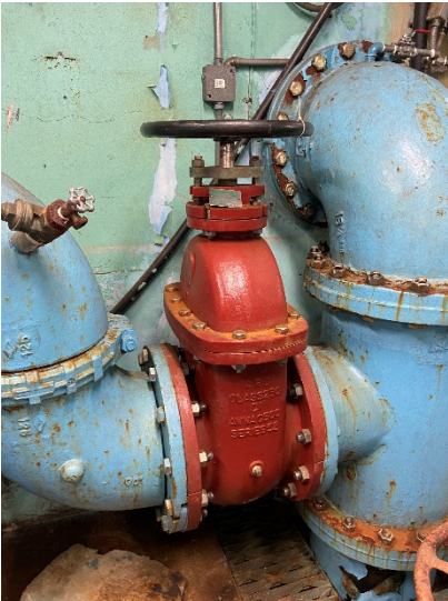
Figure 45: 12" gate valve
