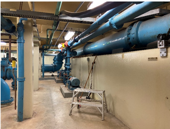
Figure 3: High Lift Pump Pipe Gallery
