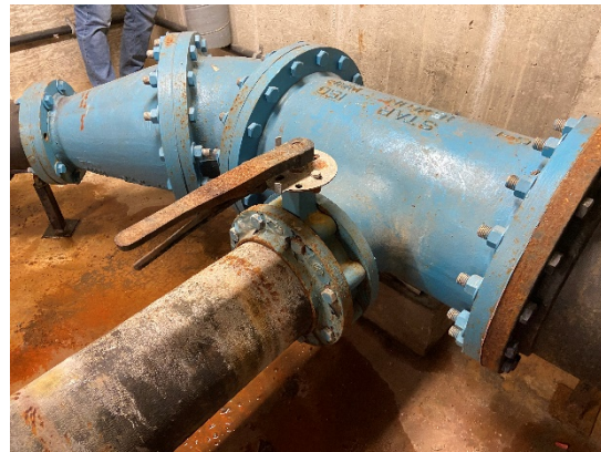
Figure 16: Butterfly valve on pump 2
