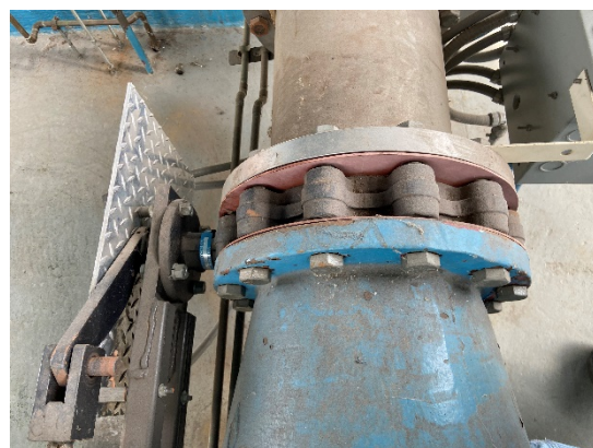
Figure 42: 10" butterfly valve on pump 5 with hydraulic controls
