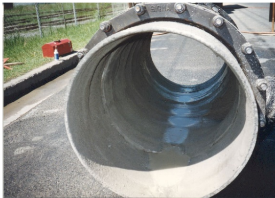
Figure 11: Cement Mortar Lined Watermain
