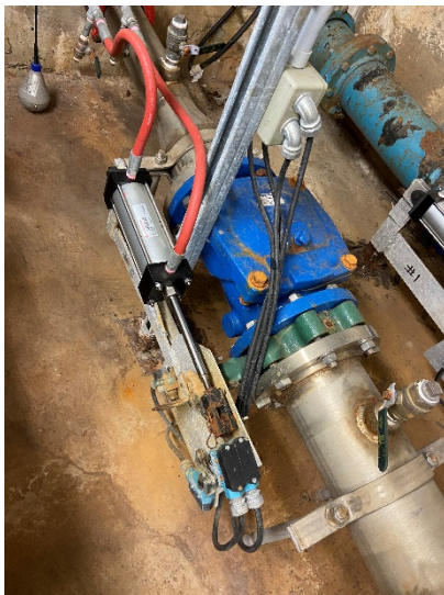
Figure 7: Butterfly and check valve on pump 2
