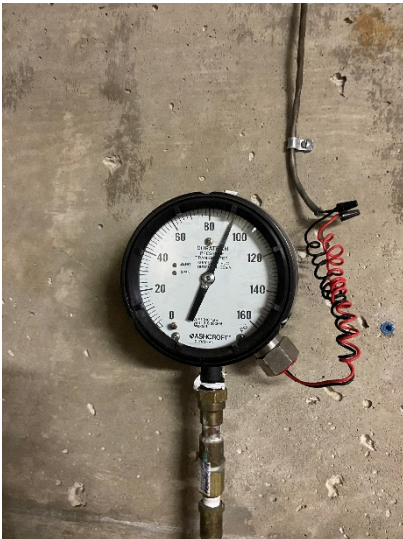
Figure 21: Discharge pressure gauge (Zone 2)
