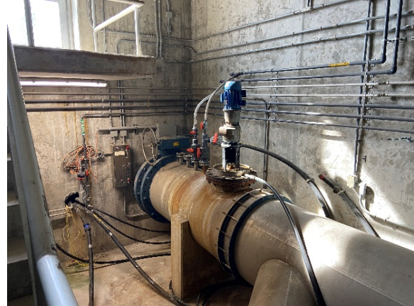
Figure 2: Raw Water Piping, Coagulant Injection Point and Mixer
