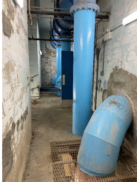
Figure 2: Intake Piping between wet well and low lift pumps
