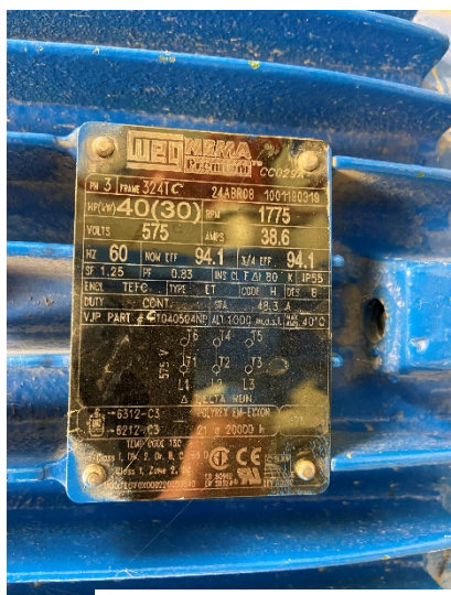
Figure 9: Label on pump 1
