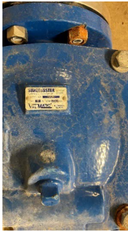
Figure 11: Label on check valve
