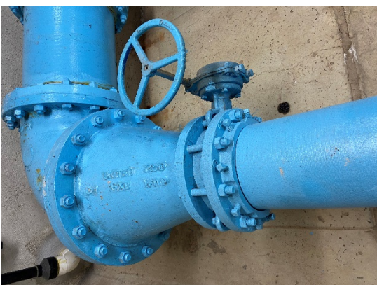
Figure 11: Butterfly valve on pump 1 (suction)
