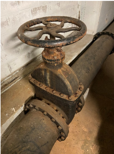
Figure 17: Zone 1 discharge gate valve
