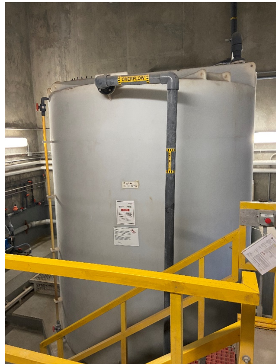
Figure 6: 25,000L Fluoride Storage Tank
