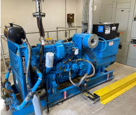
Figure 1: 192 kW generator
