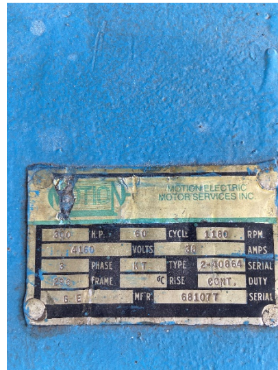
Figure 46: Label on pump 5 motor
