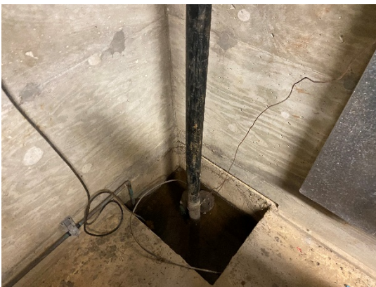
Figure 23: Sump pump
