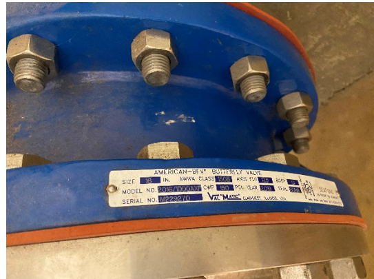
Figure 4: Label on butterfly valve
