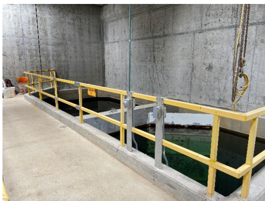
Figure 6: Floc Tanks 5B(foreground) and 5A(background)
