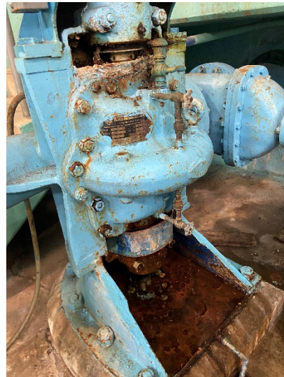
Figure 60: Pump 1 water trap
