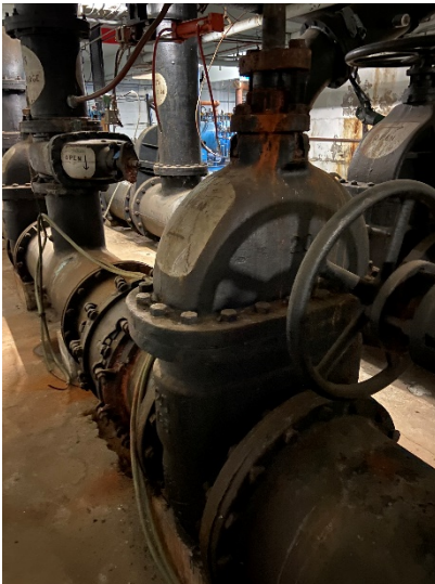
Figure 21: 20" discharge gate valve
