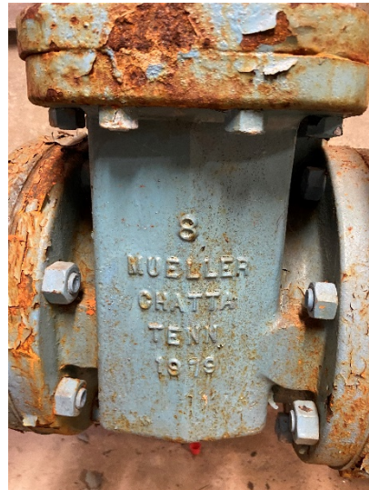
Figure 12: Gate valve
