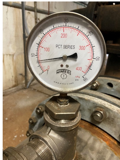
Figure 8: Suction pressure gauge
