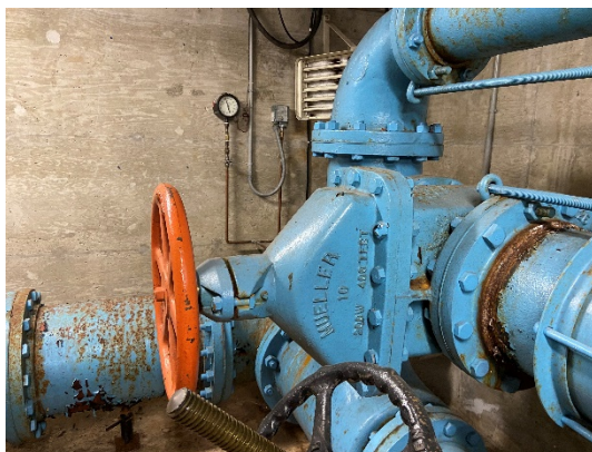
Figure 28: Gate valve on by-pass
