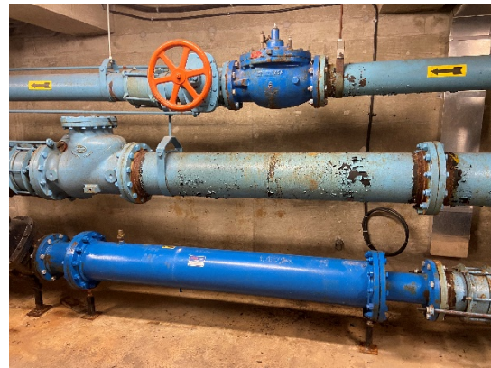
Figure 6: Pump 3, check valve and pressure reducing valve
