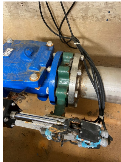
Figure 8: Butterfly and check valve on pump 1
