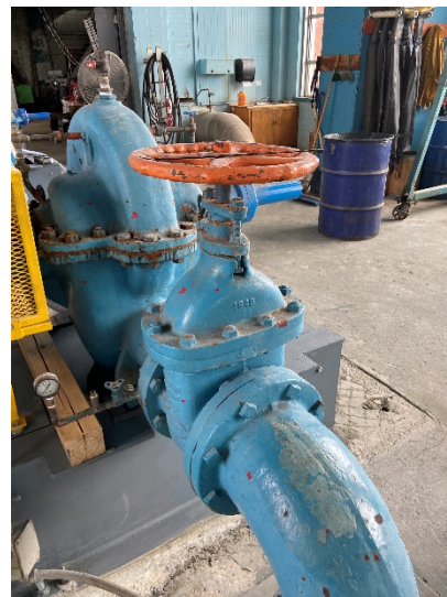
Figure 62: 8" gate valve on pump 2
