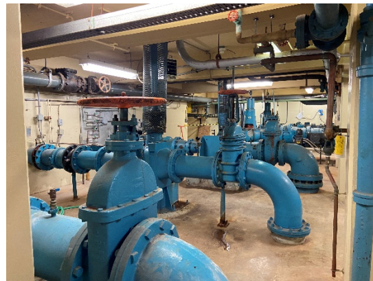
Figure 4: High Lift Pumps – Valves and Piping
