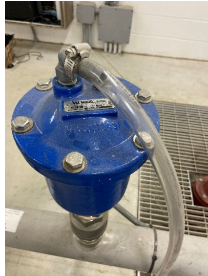
Figure 18: Suction air release valve on pressure reducing valve
