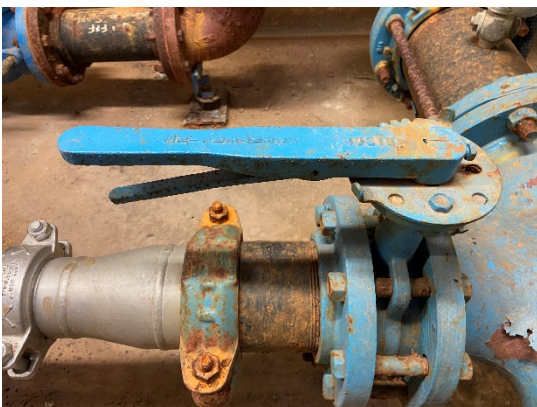
Figure 5: Butterfly control valve on pump 1
