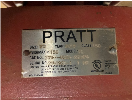
Figure 13: Label on butterfly valve
