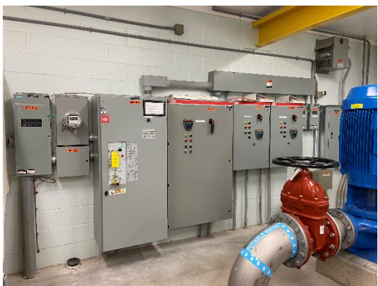
Figure 6: SCADA and electrical equipment
