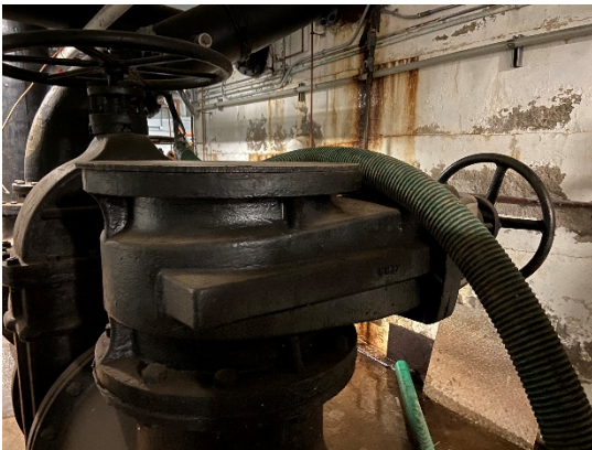
Figure 29: Out of use gate valve
