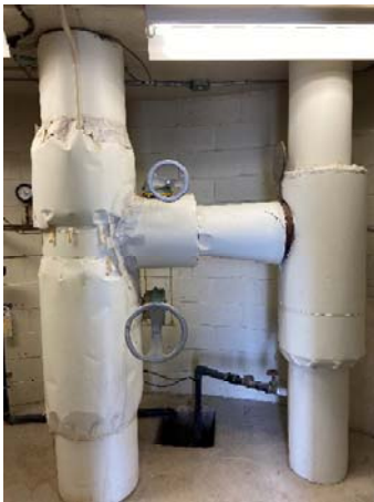
Figure 3: Two butterfly valves on 12" feed pipe and 6" overflow pipe
