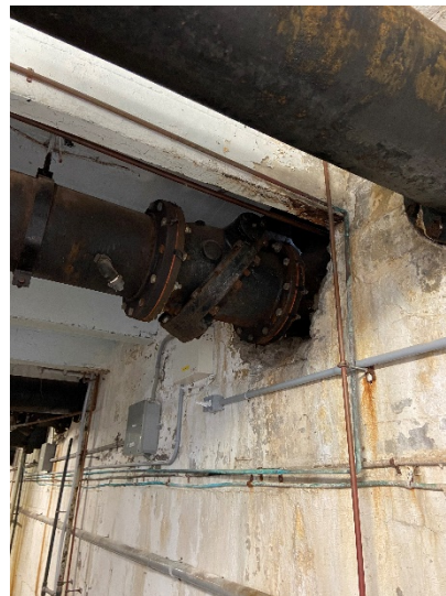
Figure 4: Pump 1 12" discharge check valve
