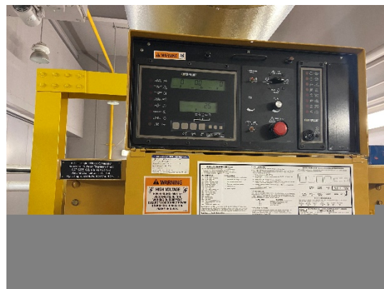
Figure 6: Generator Controls
