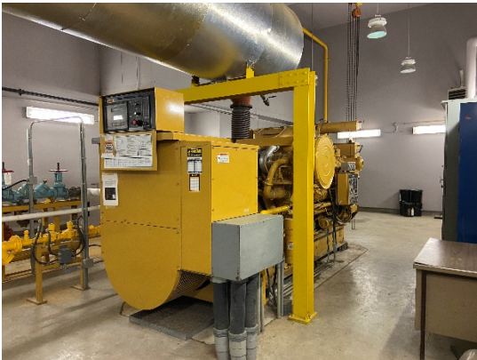
Figure 3: Motor with Gen Set
