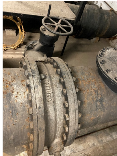
Figure 38: 30" butterfly valve
