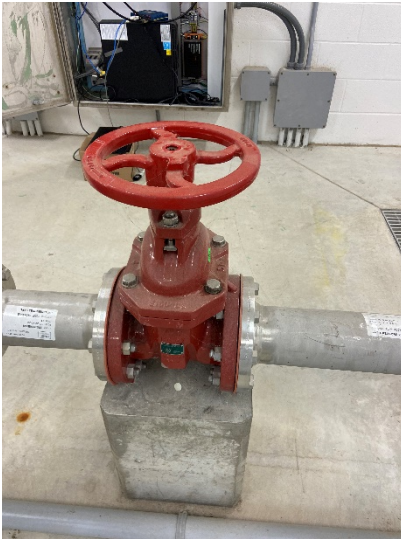
Figure 17: Suction gate valve on pressure reducing valve
