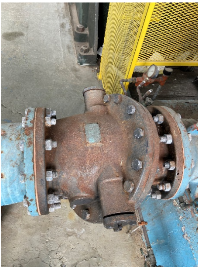
Figure 49: Pump 4 check valve
