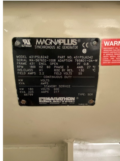
Figure 12: Label on the AC generator
