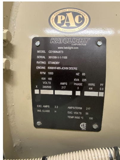
Figure 14: Label on the generator's engine
