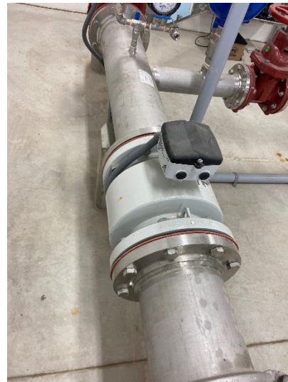
Figure 12: Flow meter
