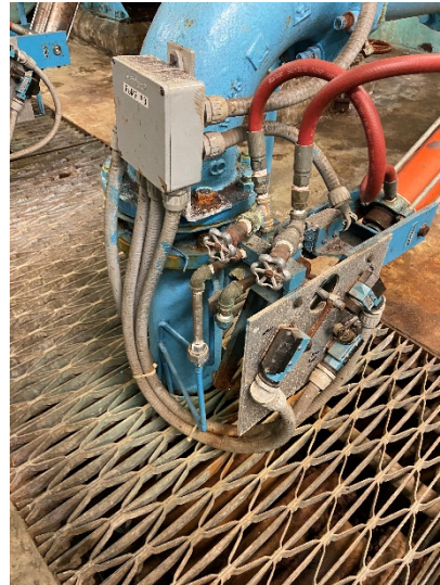
Figure 26: Hydraulic butterfly valve on pump 3
