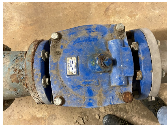
Figure 10: Swing check valve on pump 2
