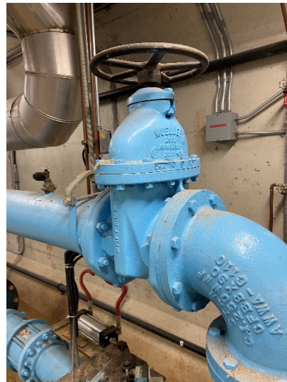
Figure 28: Discharge gate valve on pressure release valve
