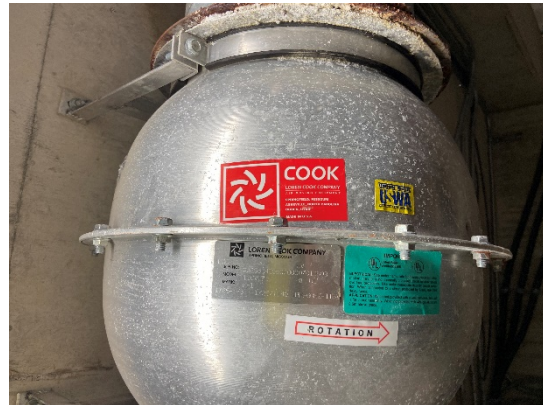
Figure 4: Exhaust Fan
