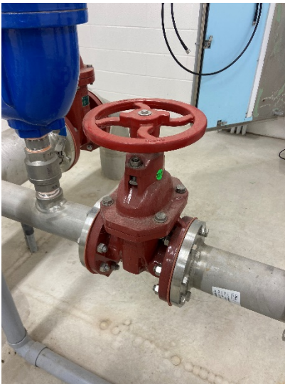
Figure 15: Discharge gate valve on pressure reducing valve
