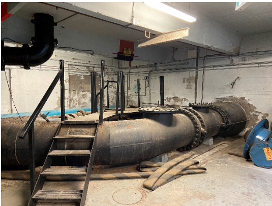
Figure 39: Suction from water treatment plant
