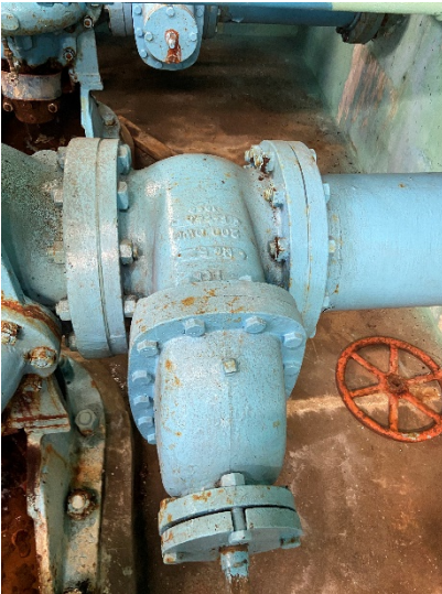
Figure 25: Check valve on pump 2
