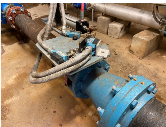
Figure 19: Reducer on pump 2
