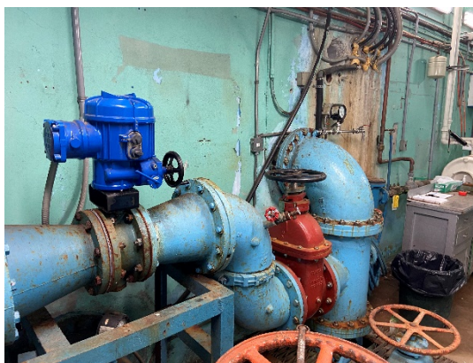
Figure 42: Butterfly valve and feed to booster pumps
