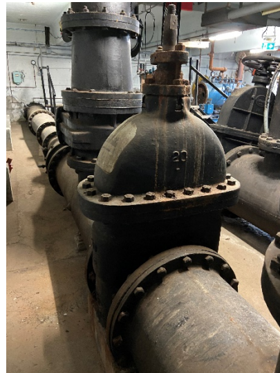
Figure 24: Zone 1 20" discharge gate valve
