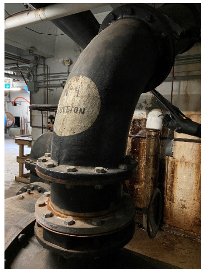
Figure 32: Pump 4 suction pipe
