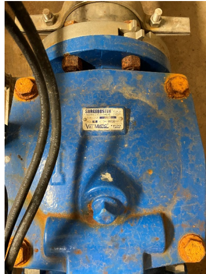
Figure 6: Check valve on pump 2
