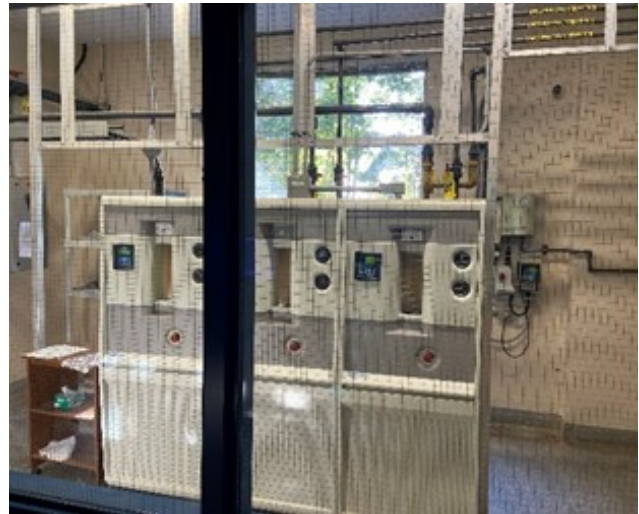
Figure 4: Chlorinator
