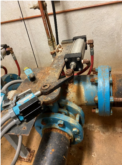
Figure 19: Butterfly valve on pump 1 (suction)
