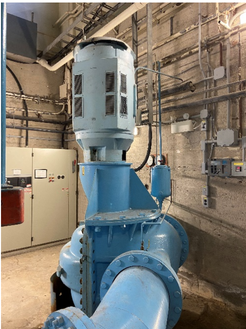
Figure 3: Electric Low Lift Pump #2
