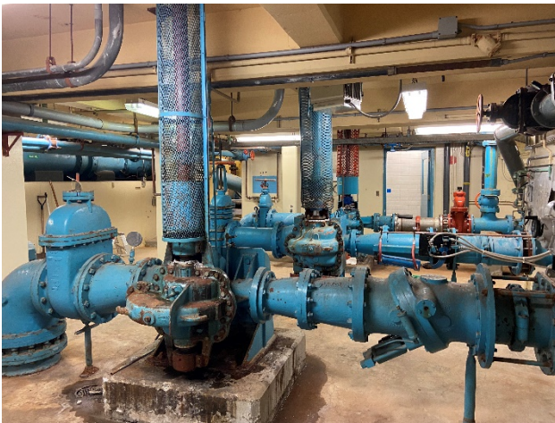
Figure 7: High Lift Pumps #1, #2 and #3
