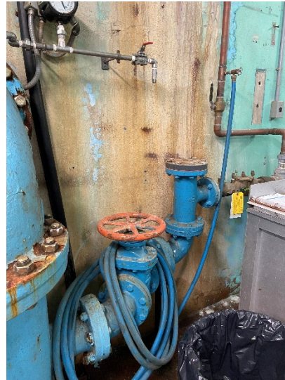
Figure 46: 4" gate valve
