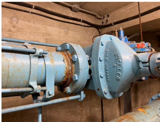
Figure 30: Gate valve on pressure reducing valve
