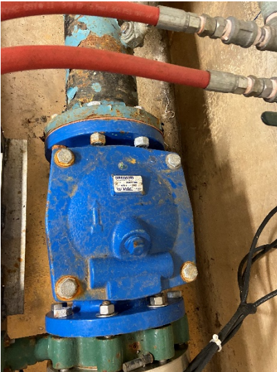
Figure 9: Check valve on pump 1
