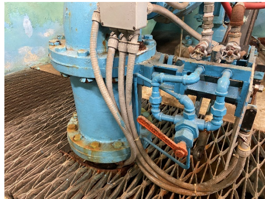
Figure 18: Hydraulic butterfly valve on pump 1
