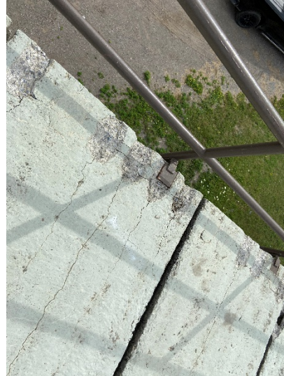
Figure 2: Cracks in concrete roof
