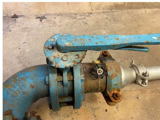
Figure 6: Butterfly control valve on pump 2
