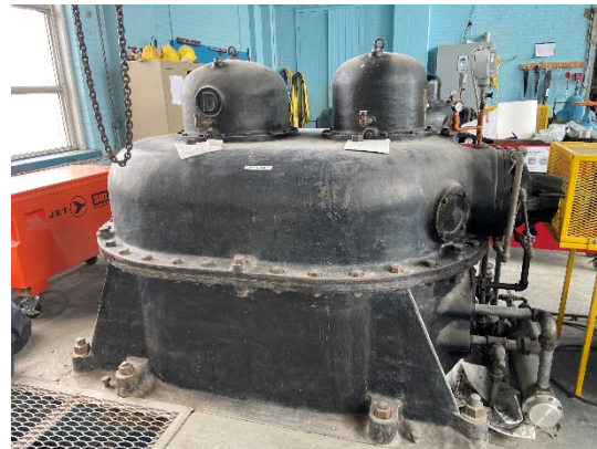
Figure 60: Gear increaser on pump 2
