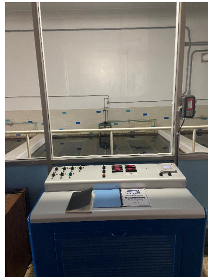
Figure 6: Filter Bed #5 and Controls
