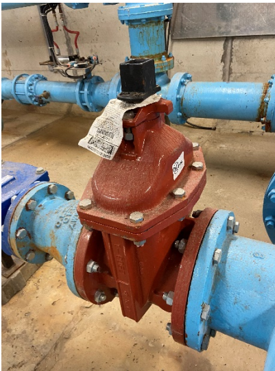
Figure 17: Gate valve on pump 2
