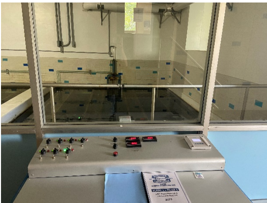
Figure 7: Filter Bed #6 and Controls
