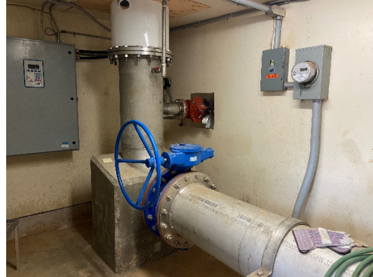
Figure 2: 16" Butterfly valve
