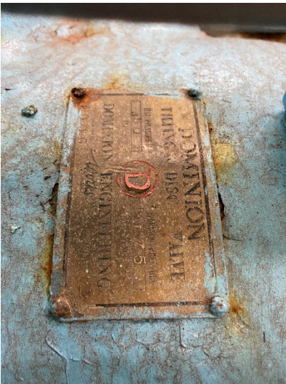
Figure 15: Label on butterfly valve
