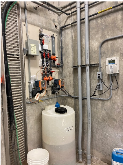
Figure 15: Dechlorination Station
