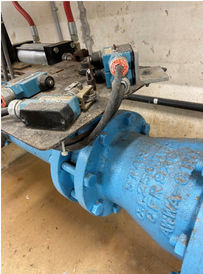
Figure 15: Butterfly valve on pump 3 (discharge)
