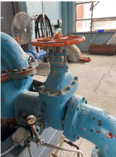
Figure 67: 8" gate valve on pump 1
