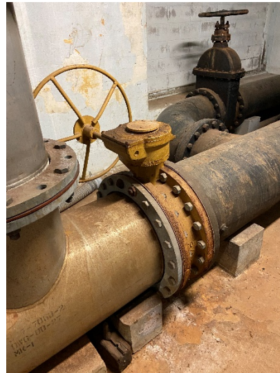
Figure 14: 20" butterfly valve
