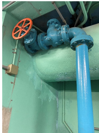
Figure 38: 4" gate and check valve
