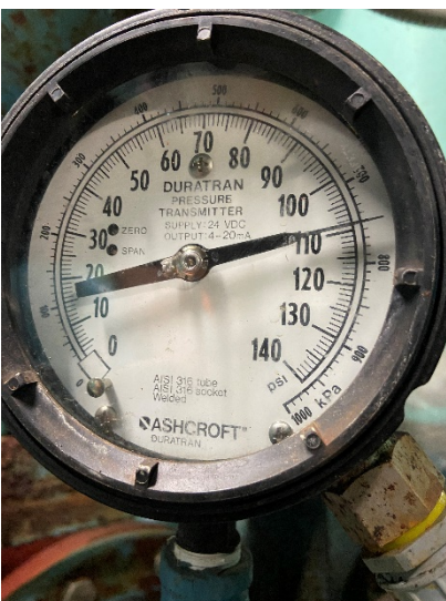
Figure 43: Pressure gauge (Discharge Pressure)
