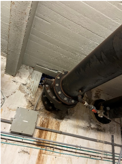
Figure 9: Pump 2 12" discharge check valve
