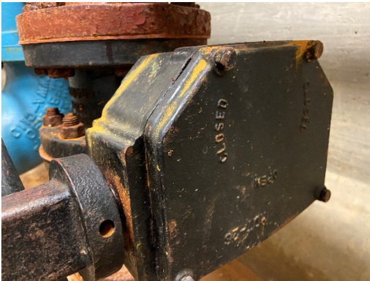
Figure 13: Butterfly valve on pressure reducing valve (suction)
