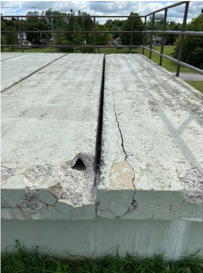
Figure 5: Cracks in concrete roof
