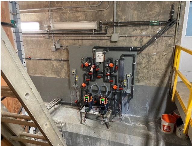
Figure 5: Sodium Hydroxide Pumps, Piping and Controls
