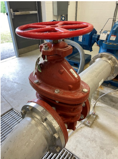
Figure 7: 8" suction gate valve on pump 2
