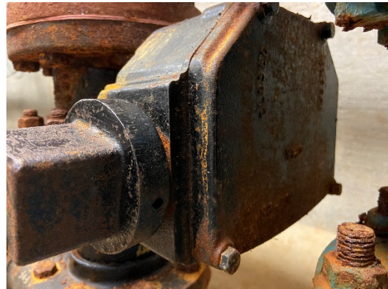
Figure 4: Butterfly valve on pressure reducing valve (discharge)
