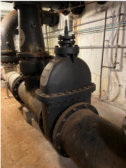
Figure 5: 20" gate valve
