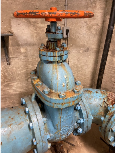
Figure 1: Gate valve in the southwest corner of the station
