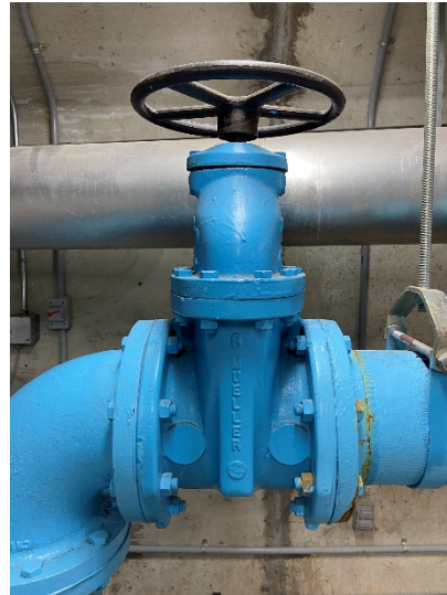
Figure 26: Gate valve on pressure release valve
