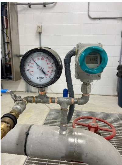
Figure 19: Suction pressure gauge (Zone 2)
