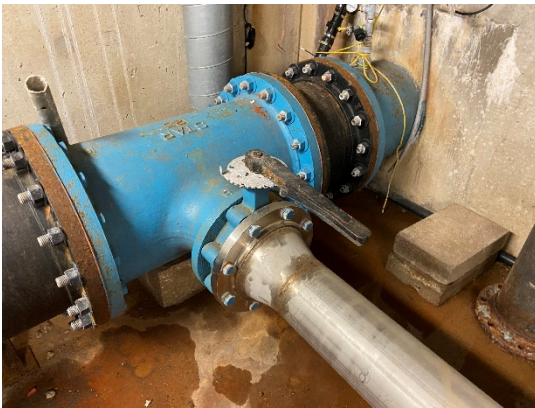
Figure 15: Butterfly valve on pump 1
