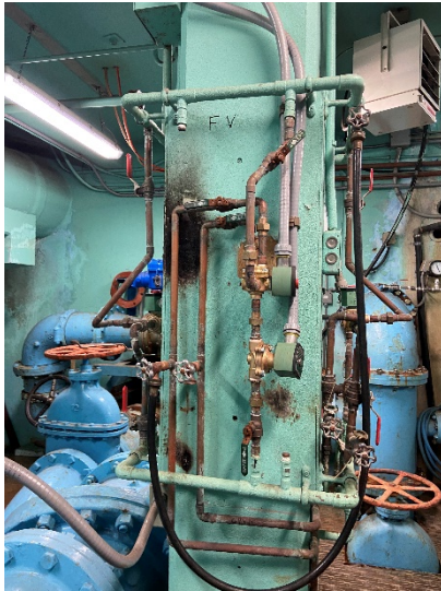
Figure 55: Butterfly valve controls
