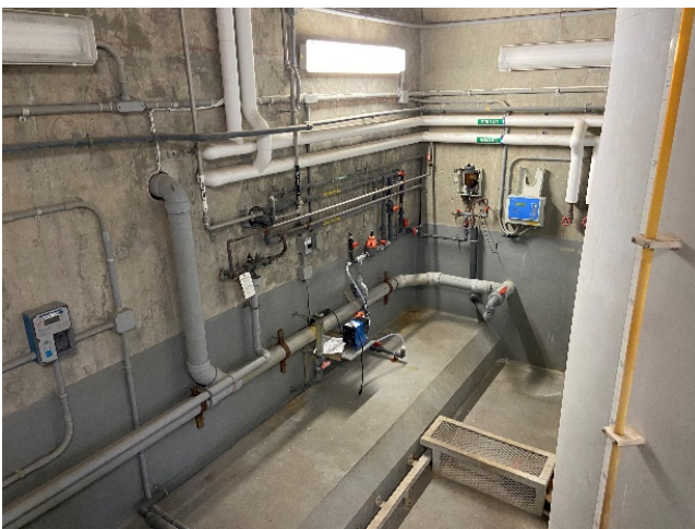
Figure 7: Fluoride Pumps, Piping and Controls
