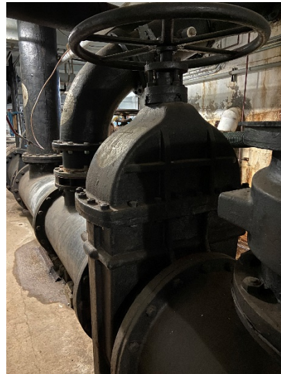
Figure 28: Suction gate valve
