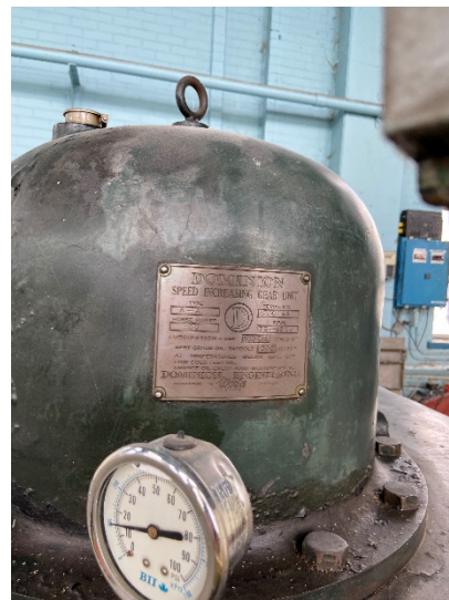
Figure 48: Label on pump 4 gear increaser
