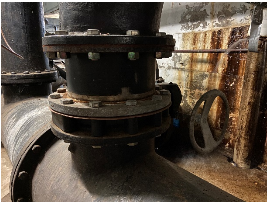
Figure 31: Pump 4 suction butterfly valve
