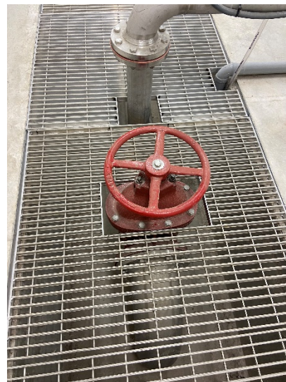
Figure 20: 8" suction gate valve
