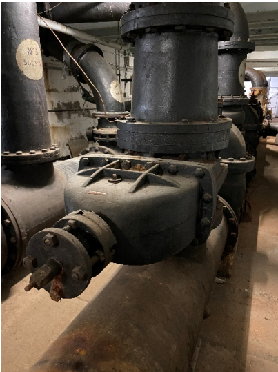
Figure 25: Pump 5 16" discharge gate valve
