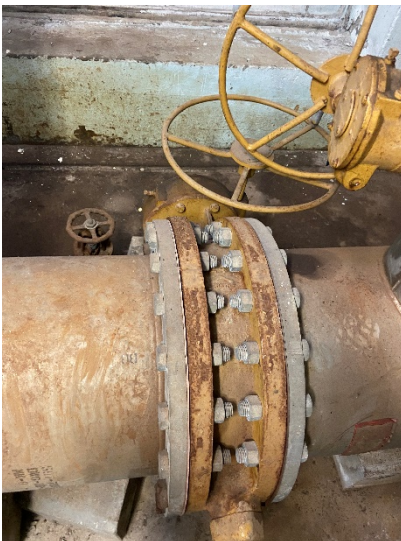
Figure 3: 24" butterfly valve
