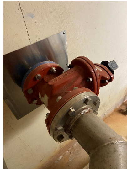
Figure 6: 4" gate valve (drain valve)
