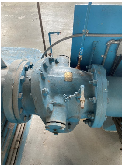
Figure 55: 10" check valve on pump 3
