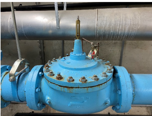
Figure 23: Pressure release valve
