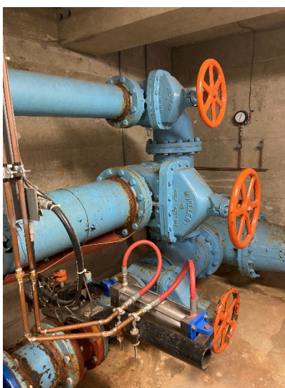
Figure 20: Gate valves
