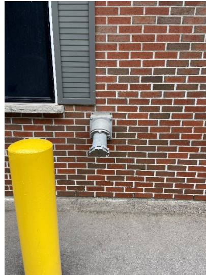
Figure 26: 240 V Receptacle (Portable Genset)
