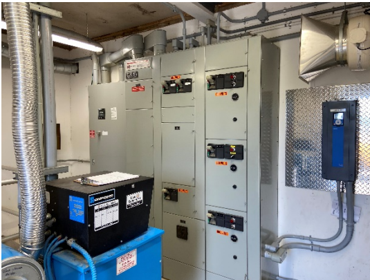
Figure 3: Electrical and SCADA equipment
