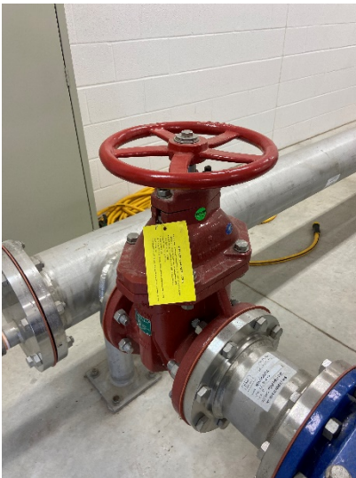
Figure 11: 6" discharge gate valve on pump 2
