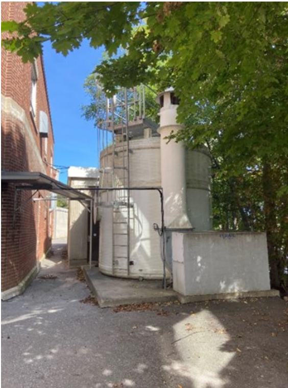
Figure 3: Chlorine Scrubber
