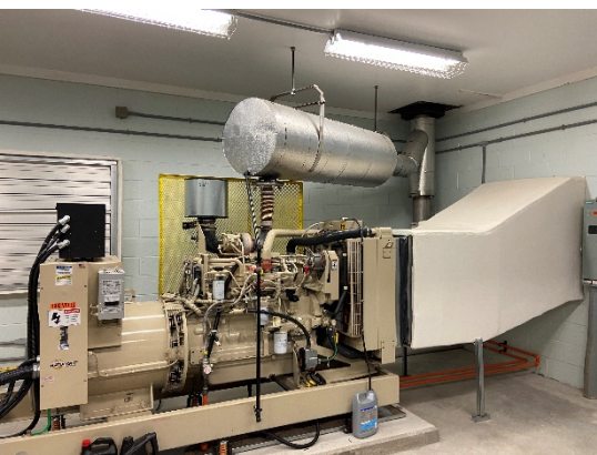
Figure 5: 180 kW Generator
