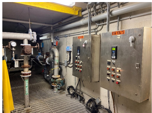
Figure 4: Sludge Tank Controls
