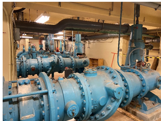
Figure 6: High Lift Pumps Check Valves
