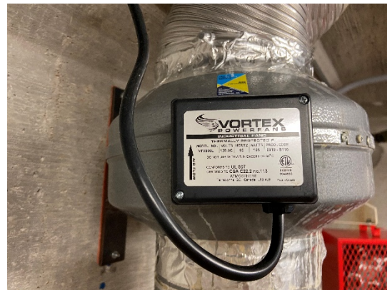
Figure 18: Exhaust Fan
