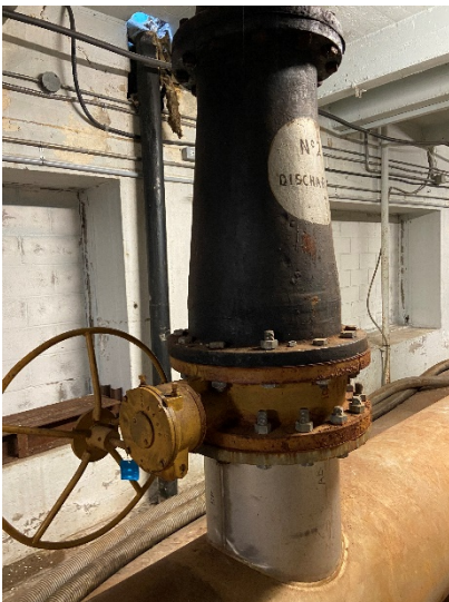
Figure 7: Pump 2 16" discharge butterfly valve
