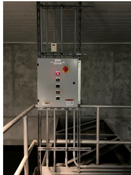
Figure 10: Thickening Tank #2 Controls
