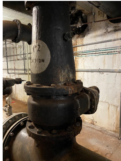
Figure 6: Pump 2 18" suction gate valve
