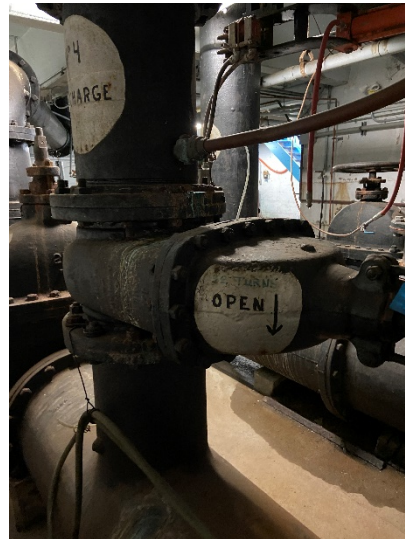
Figure 22: Pump 4 10" discharge gate valve
