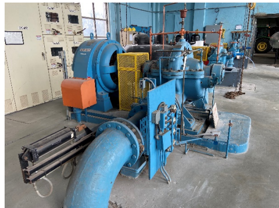
Figure 54: Pump 3 and motor
