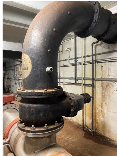
Figure 10: Pump 3 16" suction gate valve
