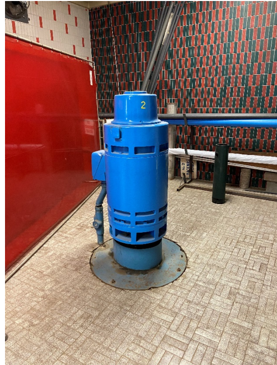
Figure 12: Backwash Electric Motor #2
