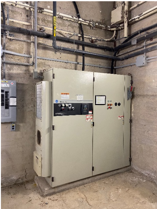
Figure 7: Low Lift Pump MC
