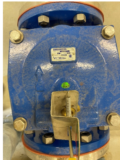
Figure 10: Check valve on pump 2
