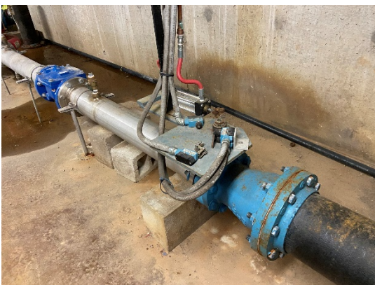
Figure 9: Check valve and reducer
