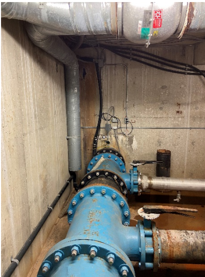
Figure 3: Discharge end of pumps, feeding back to system
