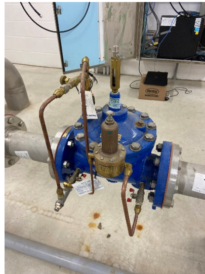
Figure 16: Pressure reducing valve
