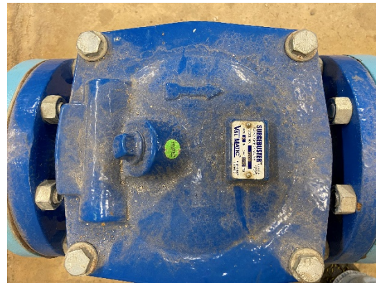
Figure 8: Check valve on pump 1
