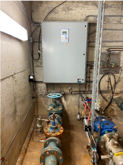
Figure 3: Pump controls in southwest corner of the station
