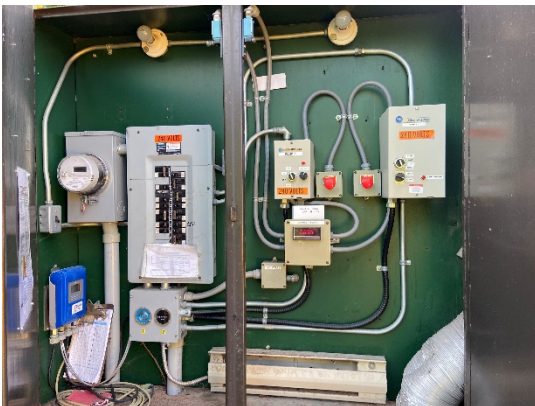
Figure 17: Electrical and SCADA box above station
