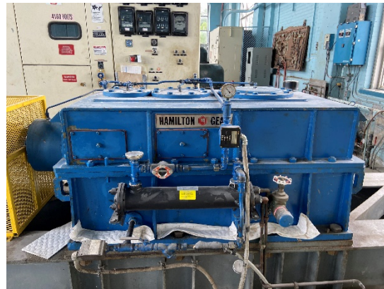
Figure 52: Generator 3 gear box
