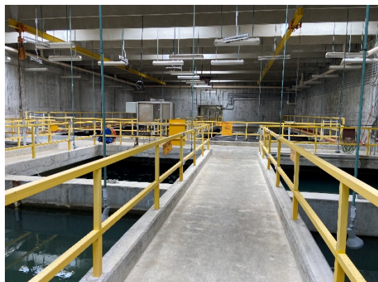
Figure 3: Floc Tanks 5/6(foreground) and Sedimentation Basins 5/6(background)
