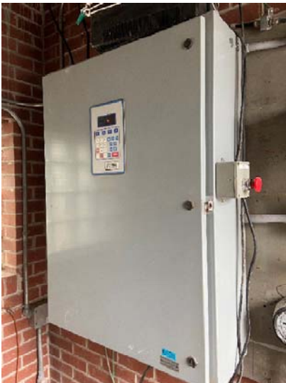
Figure 3: Electrical/SCADA cabinet
