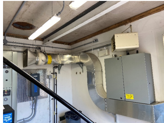
Figure 4: Ventilation system for generator
