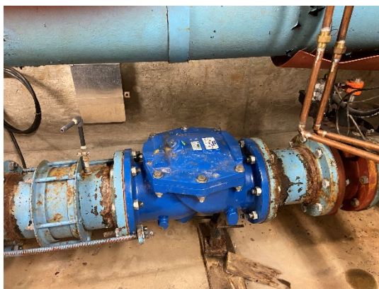
Figure 18: Check valve
