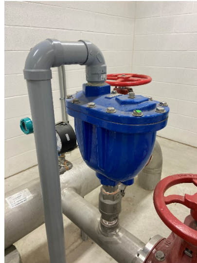
Figure 14: Air release valve
