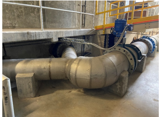
Figure 10: Post Coagulant Injection Piping to Flocculation Tanks
