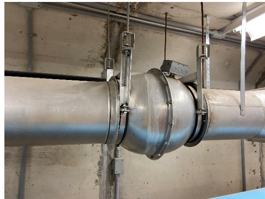
Figure 20: Exhaust Fan
