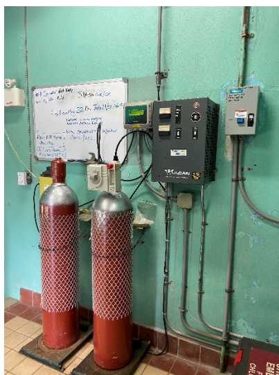
Figure 10: Chlorine injection system
