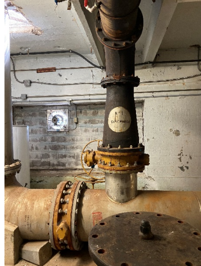
Figure 2: Pump 1 16" discharge butterfly valve
