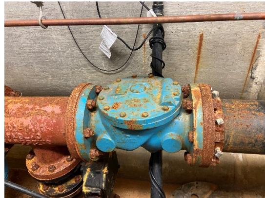
Figure 14: Check valve on by-pass
