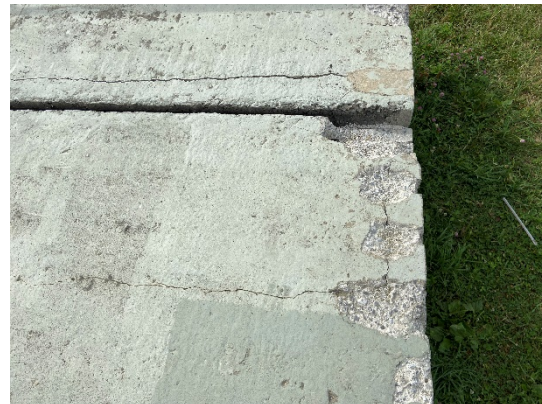
Figure 4: Cracks in concrete roof
