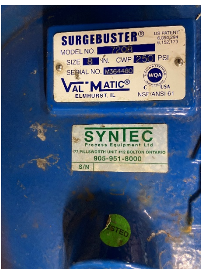
Figure 19: Label on check valve
