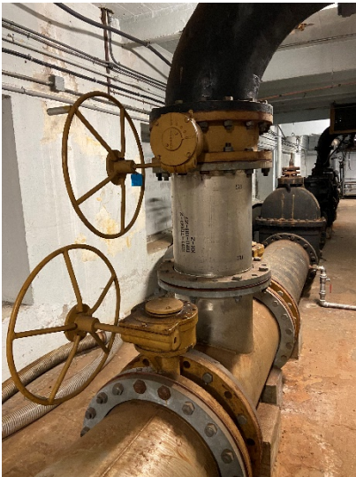
Figure 11: Pump 3 16" discharge butterfly valve
