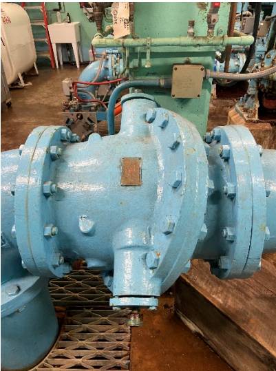
Figure 61: Pump 1 check valve
