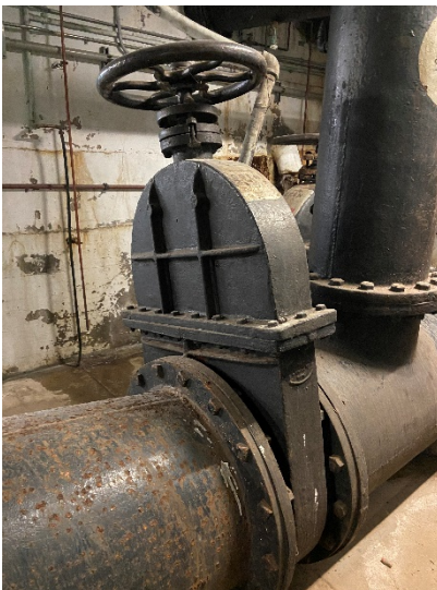
Figure 35: Suction gate valve
