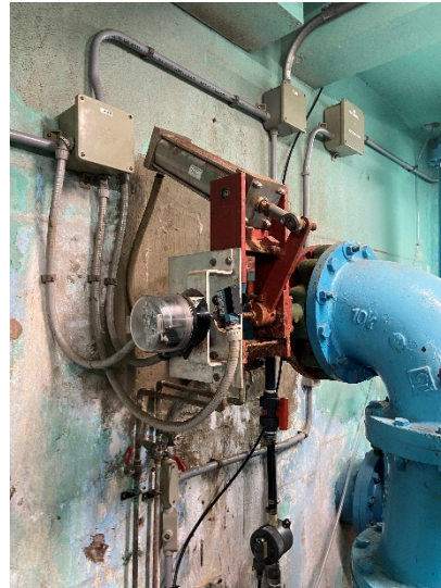
Figure 34: Hydraulic butterfly valve on reservoir feed
