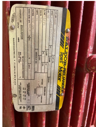
Figure 12: Label on pump 2
