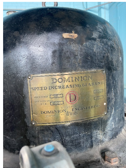
Figure 66: Label on pump 1 gear increaser
