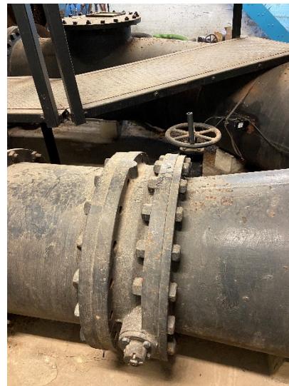
Figure 36: 24" butterfly valve
