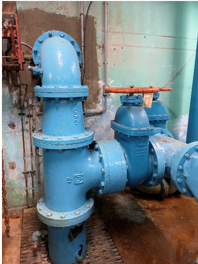
Figure 33: Gate and butterfly valves
