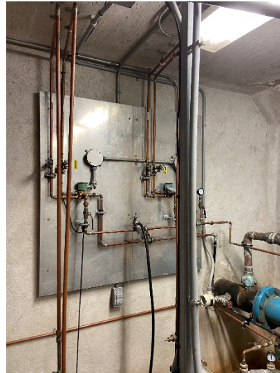
Figure 12: Automatic valve controls
