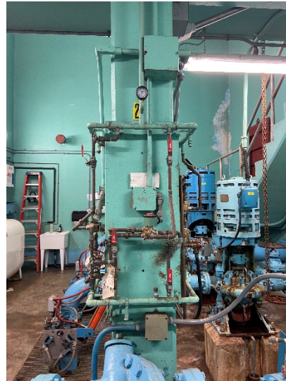
Figure 56: Butterfly valve controls
