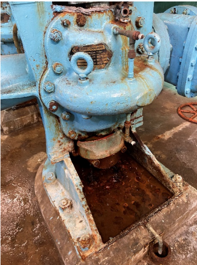
Figure 59: Pump 2 water trap
