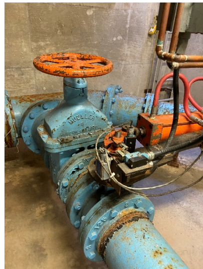
Figure 8: Gate and Butterfly valve on pump 2
