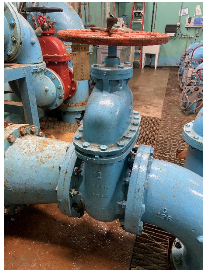
Figure 40: 12" gate valve
