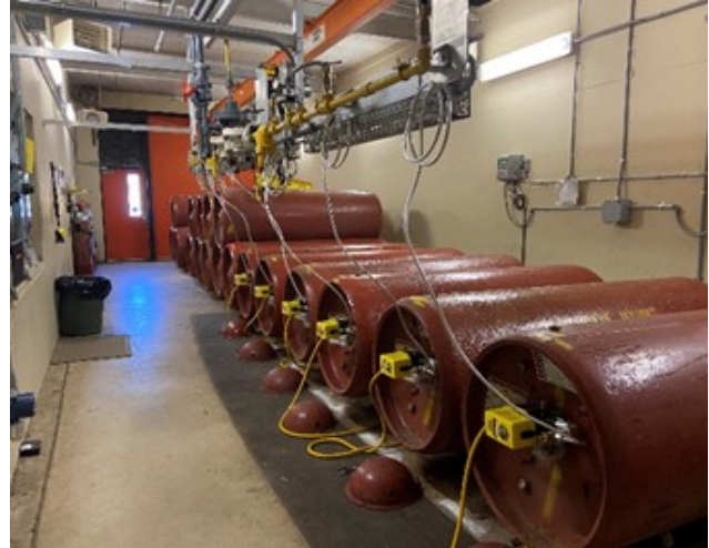
Figure 2: 18 – 1 ton Chlorine Gas Cylinders
