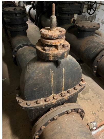
Figure 18: 20" gate valve
