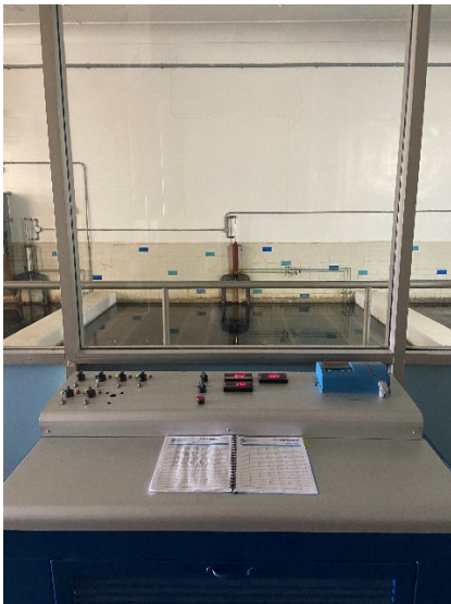
Figure 5: Filter Bed #4 and Controls
