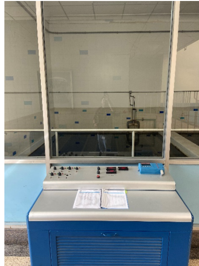
Figure 2: Filter Bed #1 and Controls
