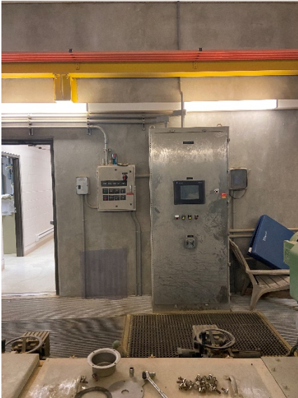
Figure 13: Centrifuge MCC
