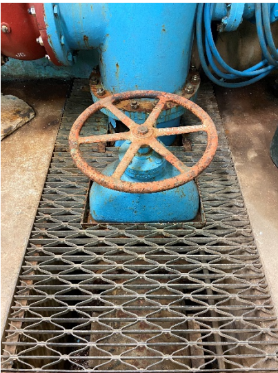
Figure 47: 18" gate valve
