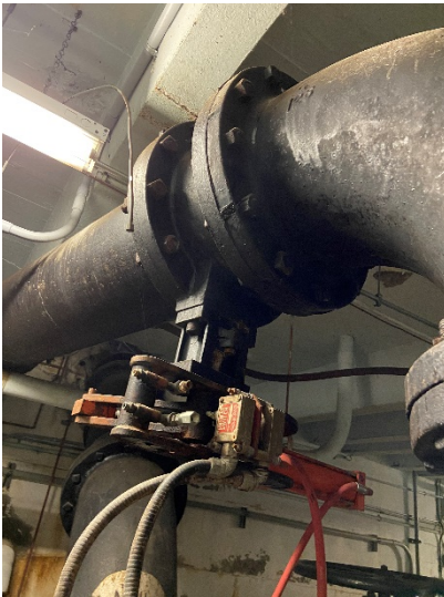
Figure 23: Pump 4 suction butterfly valve
