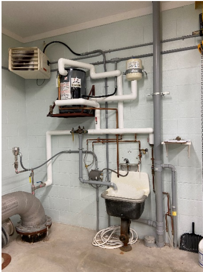
Figure 11: Electric water heater and service sink
