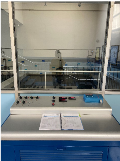
Figure 3: Filter Bed #2 and Controls
