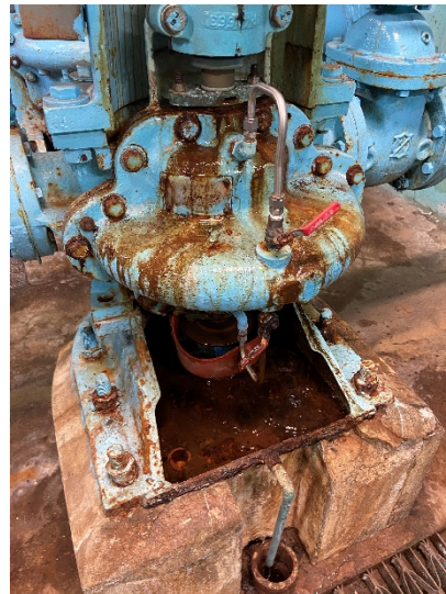
Figure 58: Pump 3 water trap
