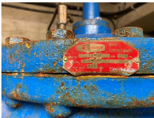
Figure 16: Label on pressure reducing valve
