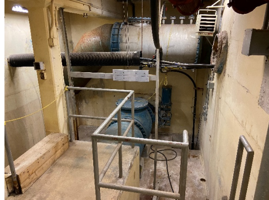
Figure 2: Chamber 'A' Backwash Piping
