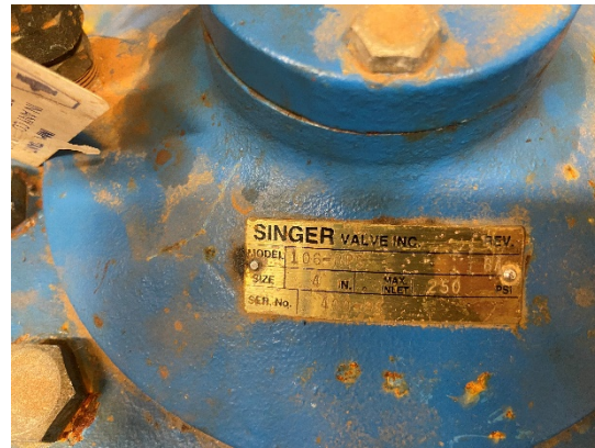
Figure 8: Label on 6" pressure reducing valve
