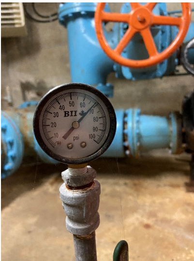
Figure 7: Discharge pressure gauge on pump 2
